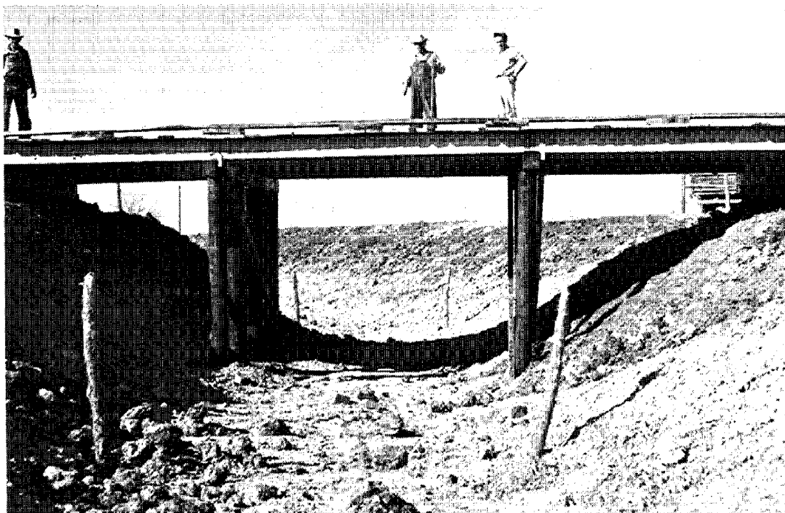
Piers are placed on each side of ditch bottom
